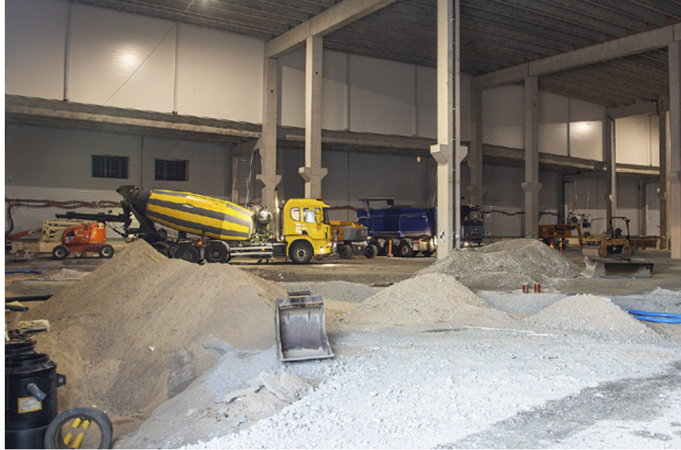
The number of construction workers at the transmission plant has averaged around 20, but the number has varied a lot according to the construction phase.
